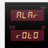
Alarm Burnig pot rotation failure
